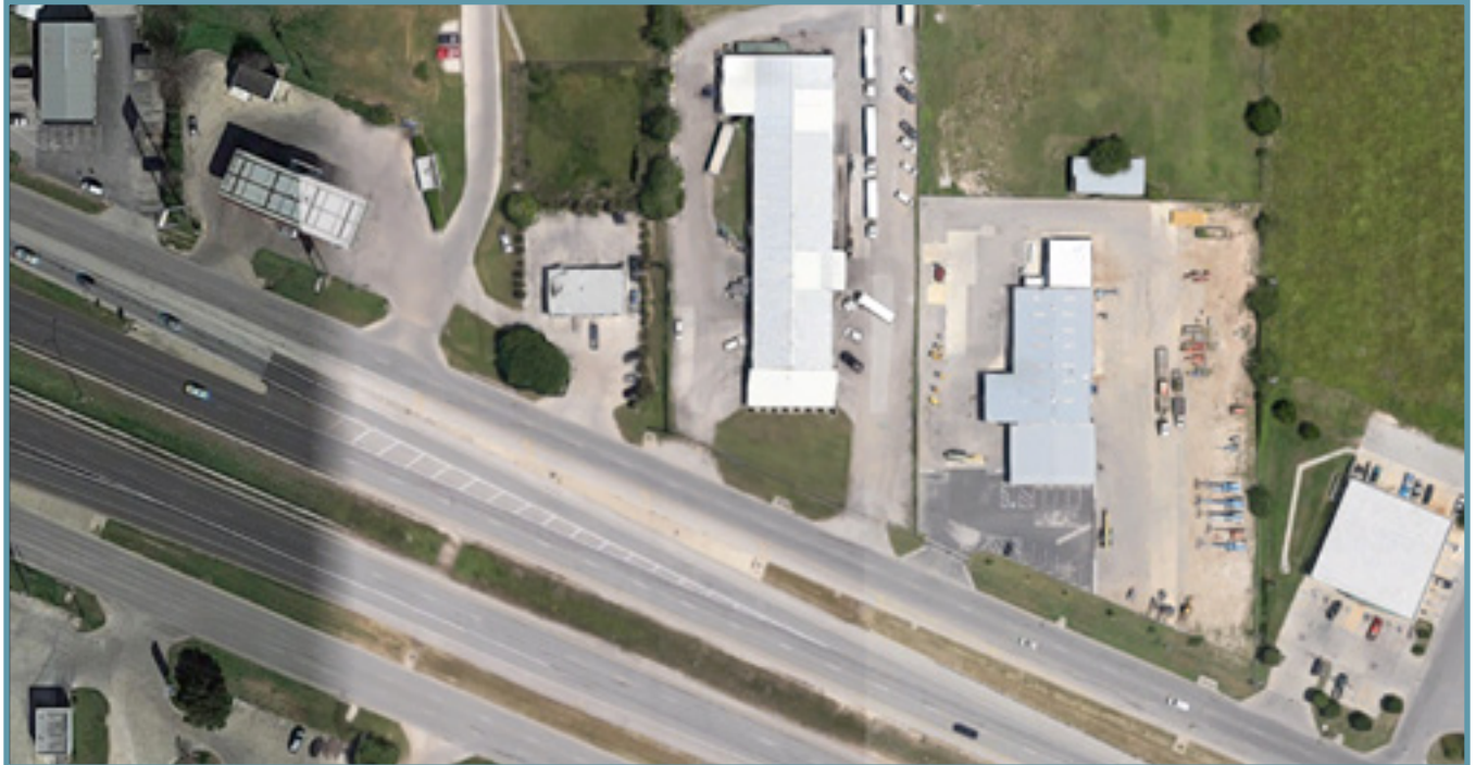
The image above illustrates nine (9) driveways cuts along an 1,100 foot segment of the SH 71/21 frontage road. Pervasive curb cuts absent cross-access and space for vehicle stacking, can severely limit roadway function.
